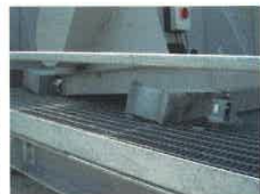
This 2 ton AC unit on the roof of Malott Hall was blown off its mountings – Mike Krings, Doug Koch/University Relations
