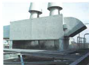
This 2 ton AC unit on the roof of Malott Hall was blown off its mountings – Mike Krings, Doug Koch/University Relations
