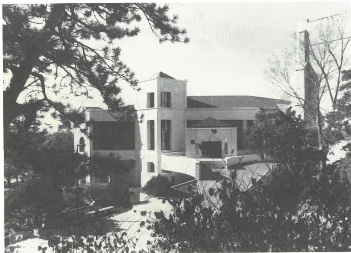
Anschutz Science Library, completed 1990.
