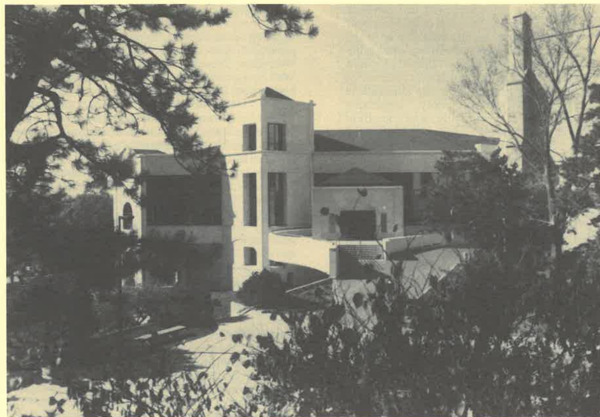
Anschutz Science Library (the SW corner of Hoch Auditorium may be seen at the right)
